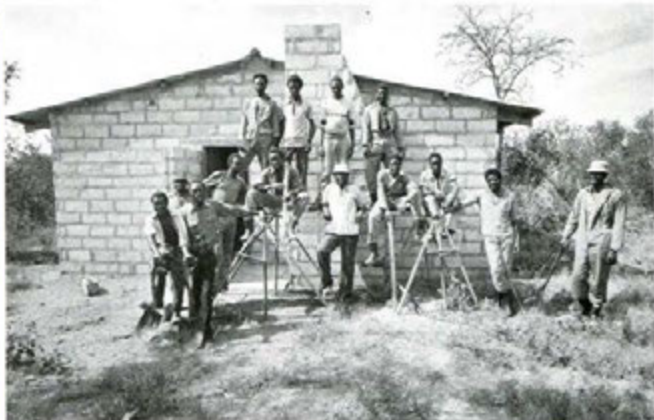
Building programme at Vukuzenzele war-disabled co-operative, near Zvishavane (Bruce Paton)
